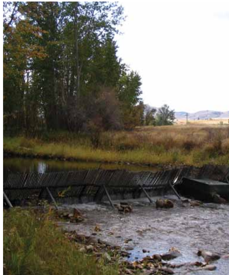
▲ PHOTO 7.6 This picket weir is set near the mouth of Red Rock Creek, Red Rock Lakes National Wildlife Refuge, Montana, looking upstream. Downstream migrating fish would be funneled into the trap in the center foreground whereas upstream migrants would be diverted to the trap on the right. The weir is made of closely spaced aluminum conduit and is held in place with metal fence posts. (Ryan Harnish)
