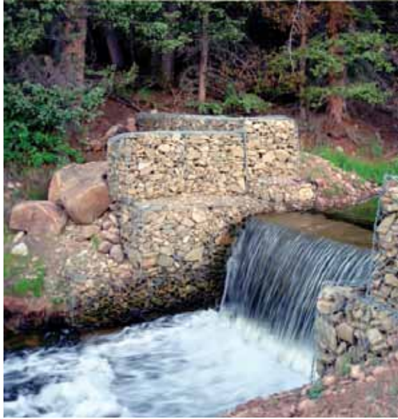
▲ PHOTOS 7.10 (left) Restoration of native fish populations is increasingly important for ecosystem management and to conform to the Endangered Species Act. Fishery biologists can isolate reaches by constructing artificial barriers to curtail upstream migration of nonnative species. 7.10 (right) A toxic chemical is introduced to reaches of streams to poison nonnative species so biologists can restore the native population. Although the chemical is destructive to the stream ecology, systems typically repair themselves in a short time. (Peter Brown)
