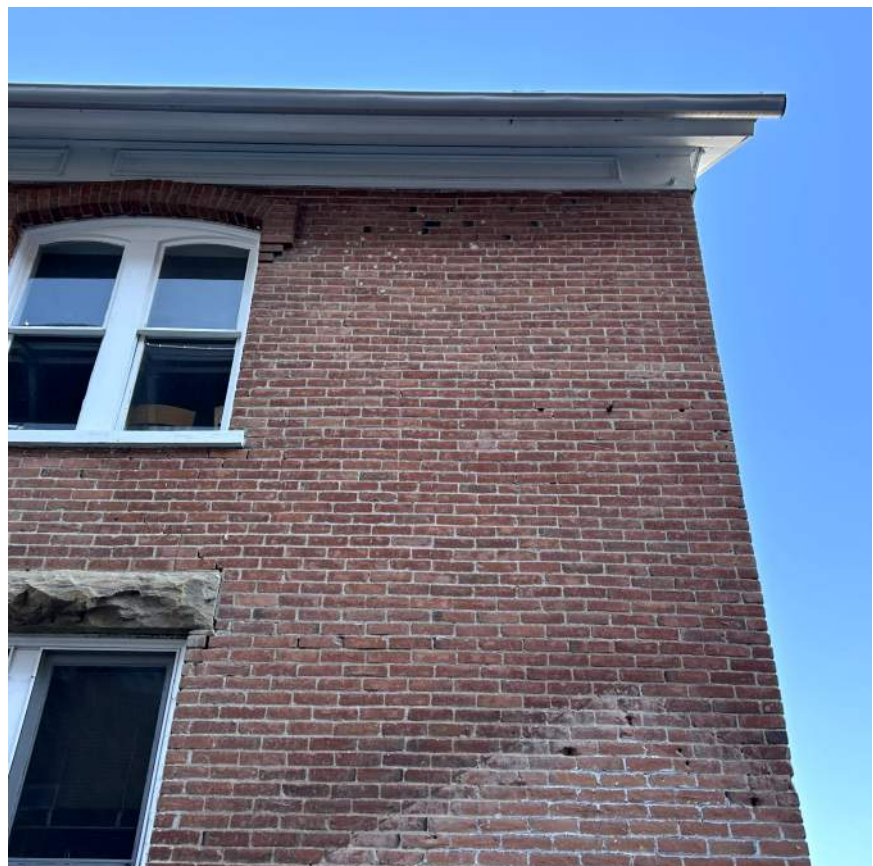
3 SOUTH DETAIL PHOTO 3 A2.4a 1 1/2" = 1'-0"
