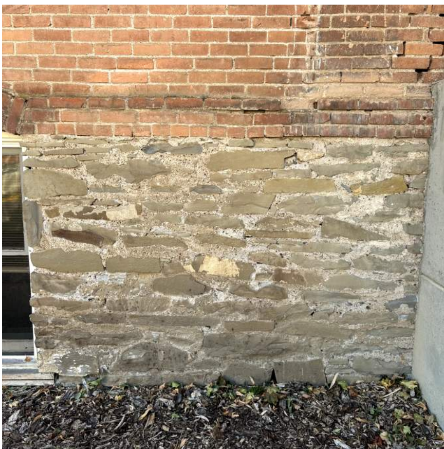
10 NORTH DETAIL PHOTO 10
