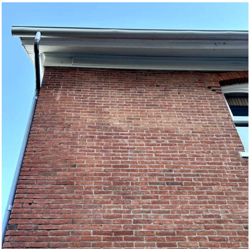
13 SOUTH DETAIL PHOTO 13 A2.4a 1 1/2" = 1'-0"
