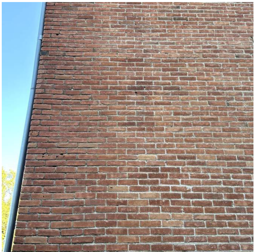
14 SOUTH DETAIL PHOTO 14 A2.4a 1 1/2" = 1'-0"
