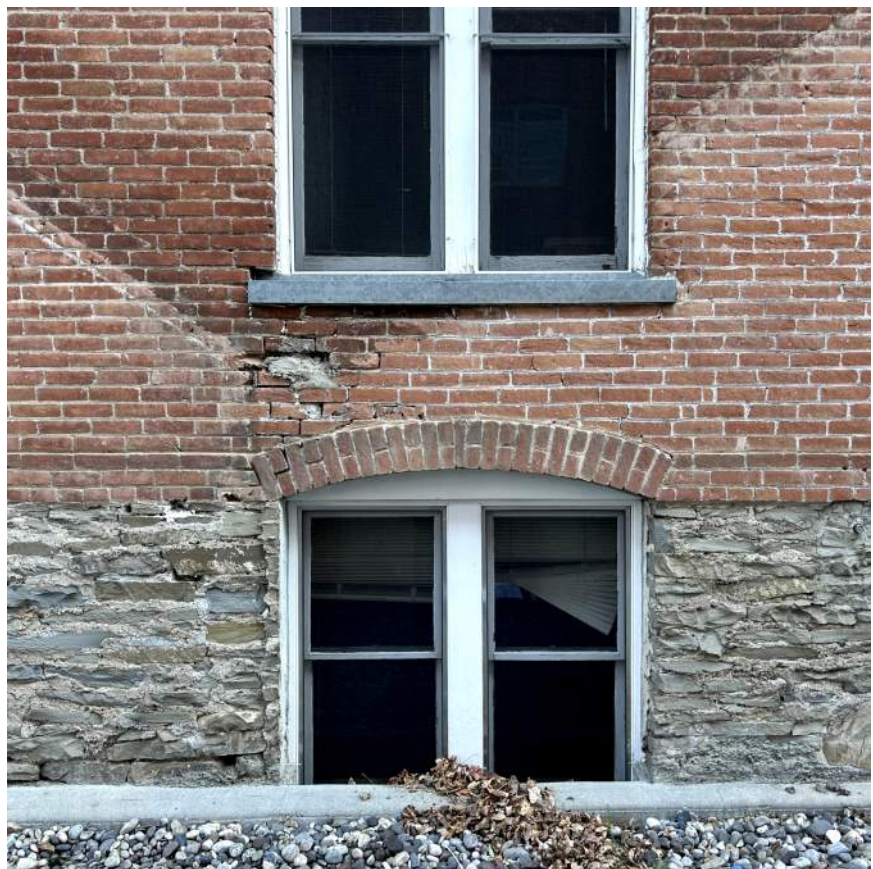
6 SOUTH DETAIL PHOTO 6 A2.4a 1 1/2" = 1'-0"
