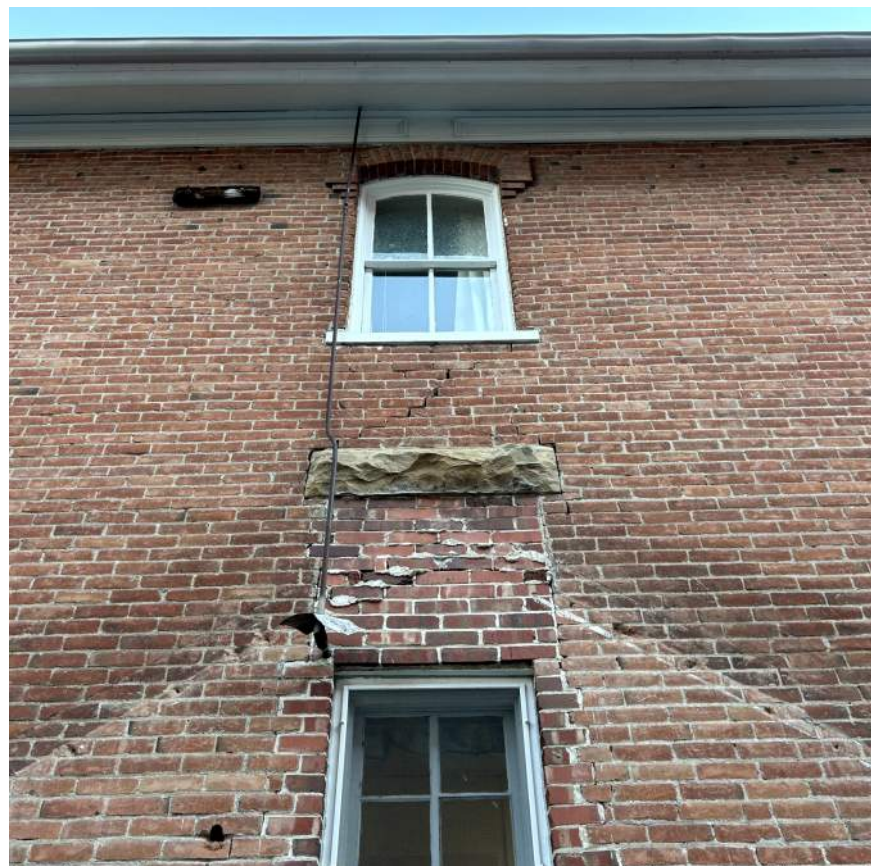
8 SOUTH DETAIL PHOTO 8 A2.4a 1 1/2" = 1'-0"
