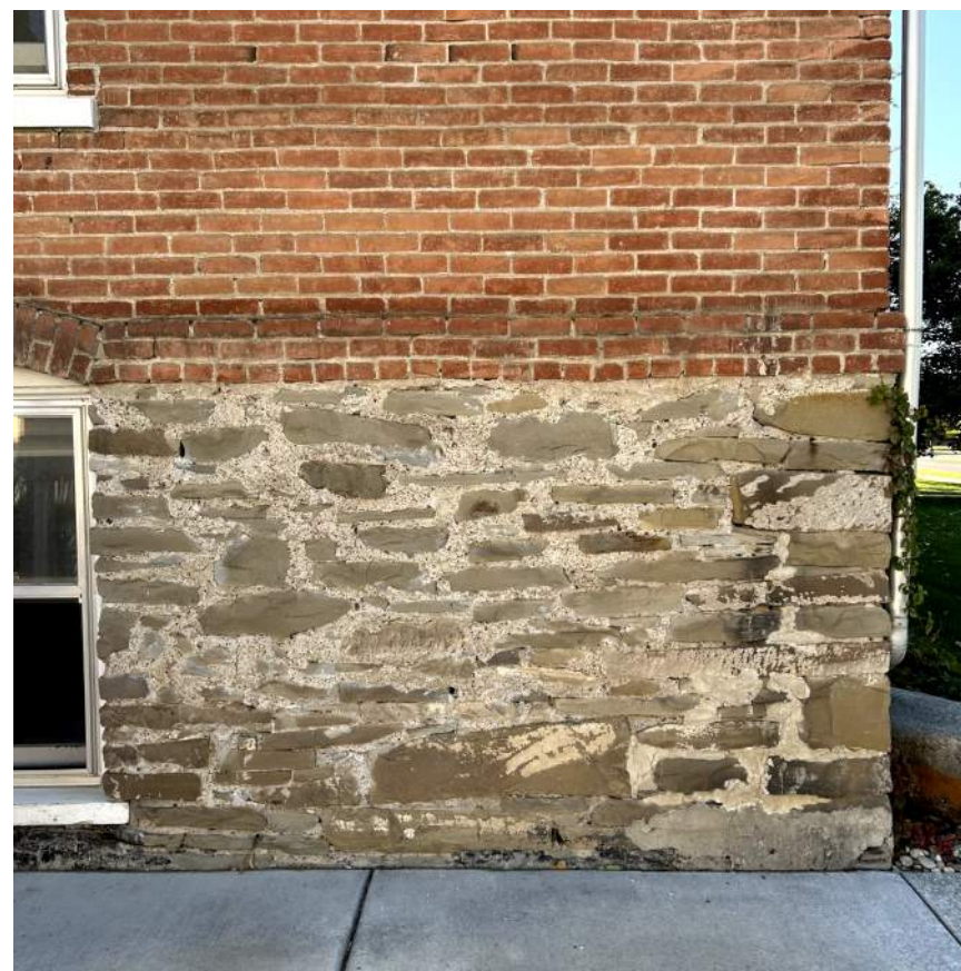
3 NORTH DETAIL PHOTO 3
