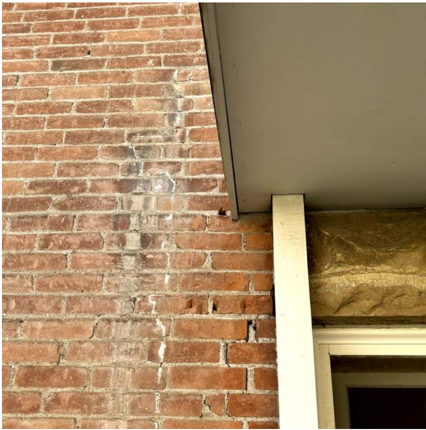
8 NORTH DETAIL PHOTO 8
