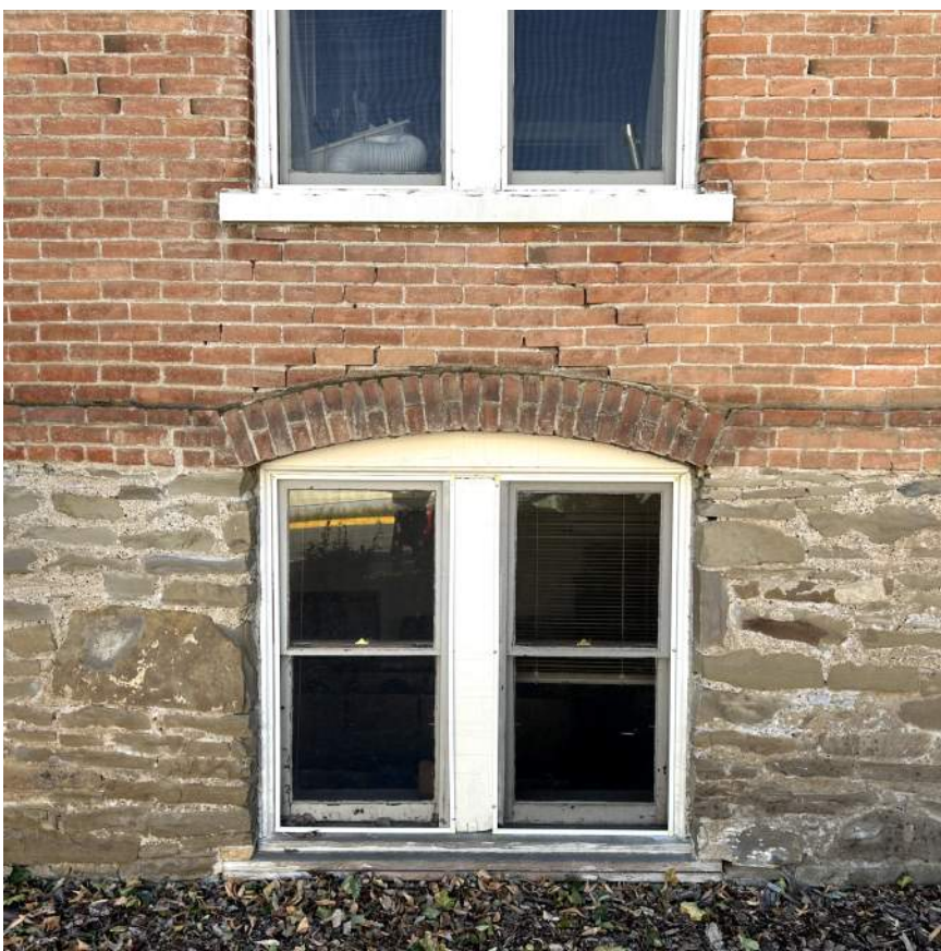
12 NORTH DETAIL PHOTO 12
