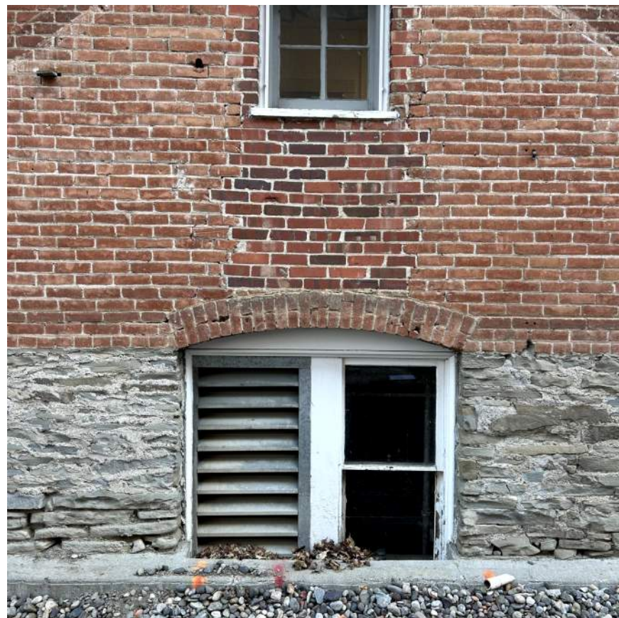
9 SOUTH DETAIL PHOTO 9 A2.4a 1 1/2" = 1'-0"
