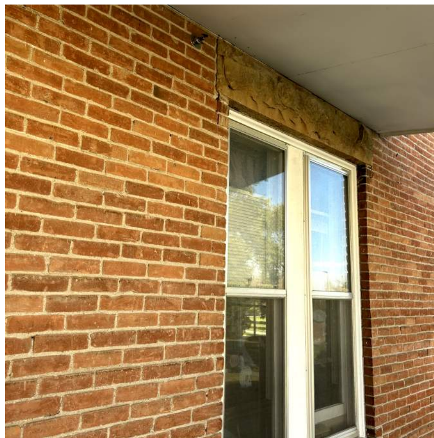
4 NORTH DETAIL PHOTO 4
