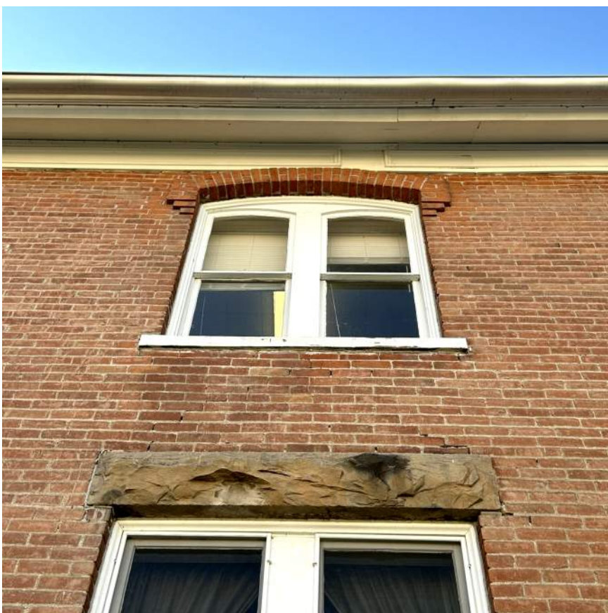
11 NORTH DETAIL PHOTO 11
