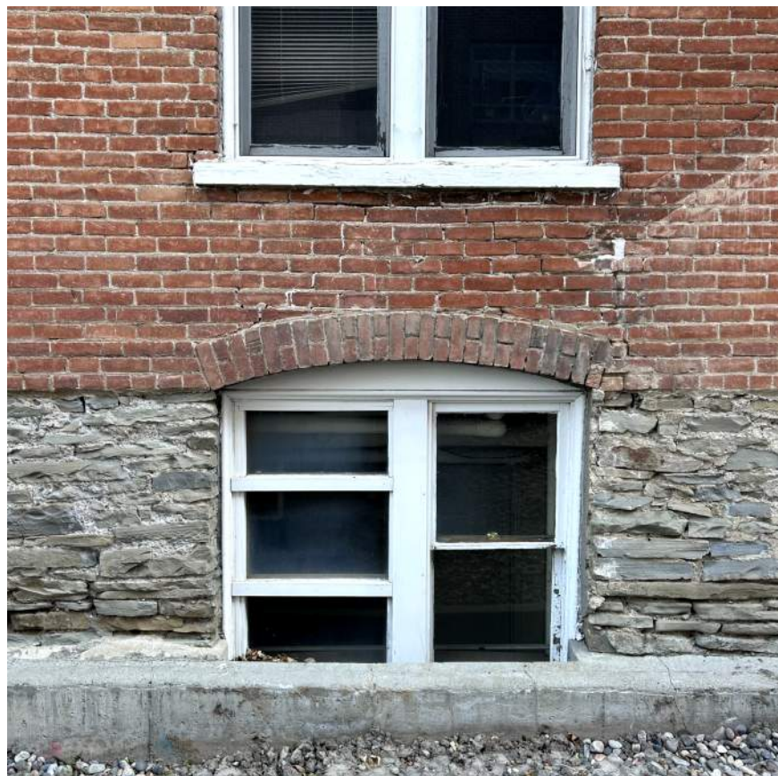
12 SOUTH DETAIL PHOTO 12 A2.4a 1 1/2" = 1'-0"
