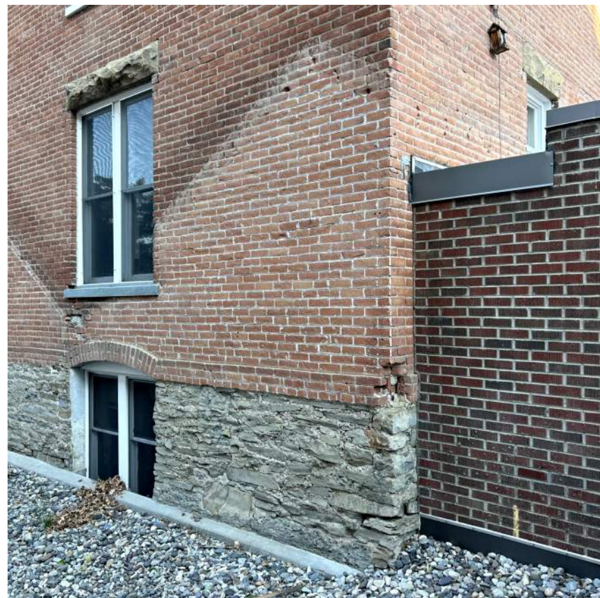
2 SOUTH DETAIL PHOTO 2 A2.4a 1 1/2" = 1'-0"
