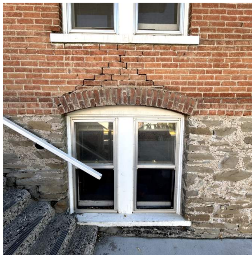
5 NORTH DETAIL PHOTO 5
