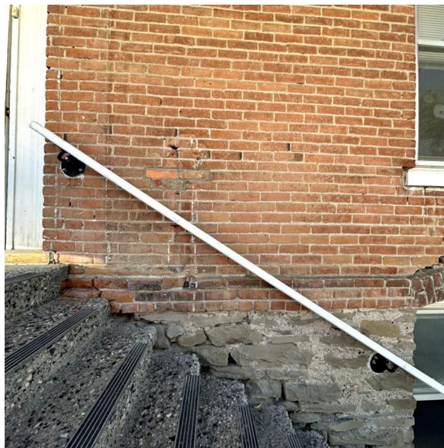
7 NORTH DETAIL PHOTO 7
